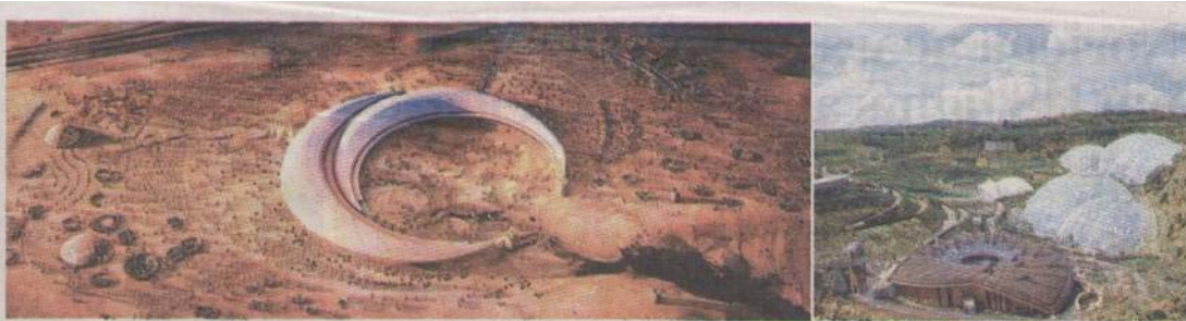
An artist's impression of the planned 'evolutionary gardens' near Riyadh in Saudi Arabia. They will be five times the size of the Eden Project biodomes near St Austell in Cornwall, right
